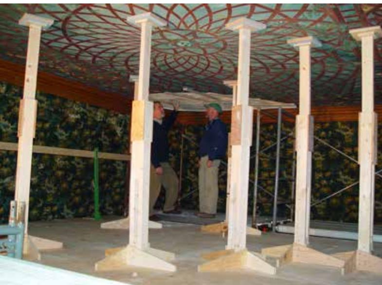
Figure 15 Jacks secure unstable ceiling.
