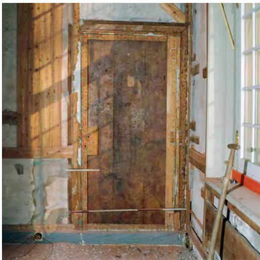
Figure 4a-b A grained door discovered in Trompenburg (c.1675), 's-Graveland. Photo A.J. van der Wal, Collection RCE, object nr. 507.931, 2003.
